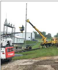
the transmission line into the substation is being replaced. Inside the substation, CRMU will be replacing the gang-operated air-break switches, the fused knife switches, along with installing a new secondary riser structure and metering cabinet.
